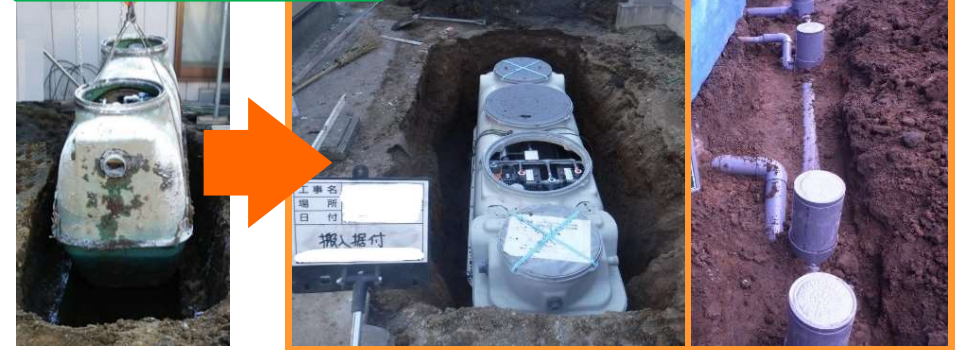
Old type removal Current type installation Piping works
